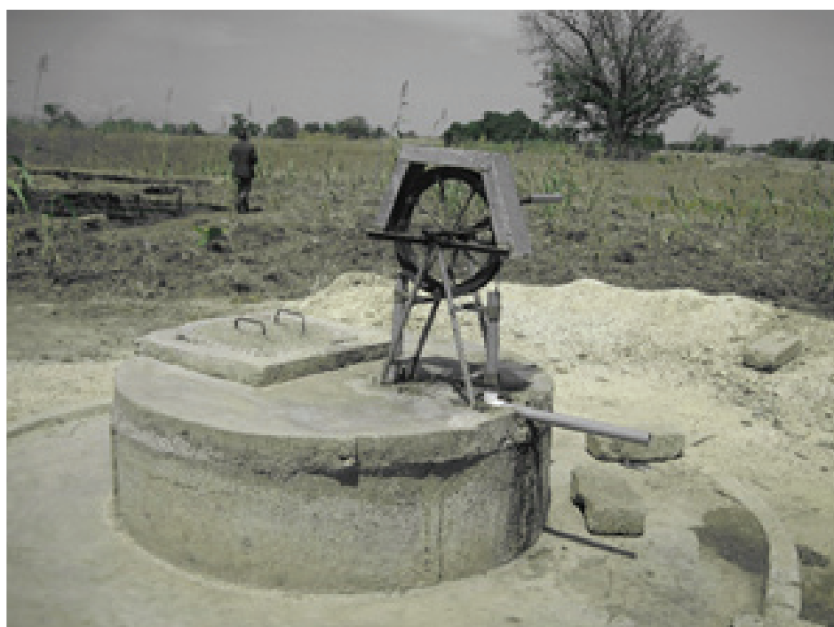
Wells fitted with rope and soka pumps have been made available at all project farm sites to make water readily available to aid dry season gardening
